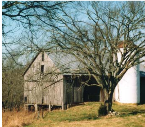
Homeplace barn said to have been built with lumber from the 1863 Green River Bridge.
